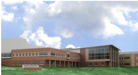
ELKHORN SOUTH HIGH SCHOOL 20303 BLUE SAGE PARKWAY 402-289-0616 PRINCIPAL: MARK KALVODA
